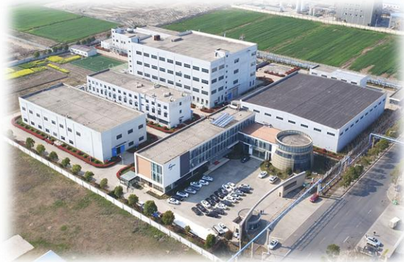
Nantong Catalyst Factory
